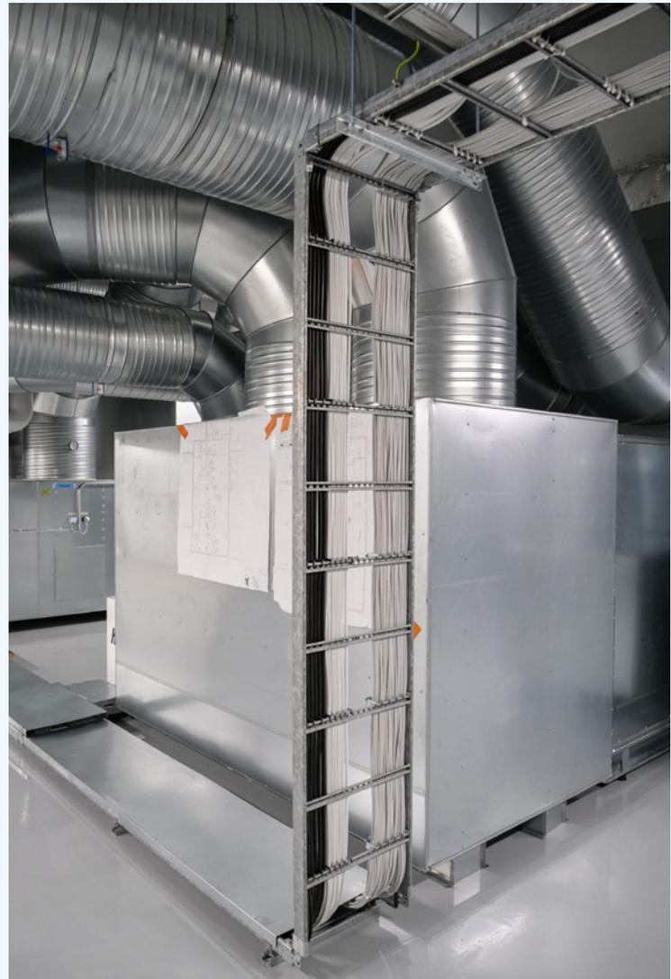
The joints in the chart create a sufficient electrical joint, which eliminates the need to install a separate grounding wire between trays.
