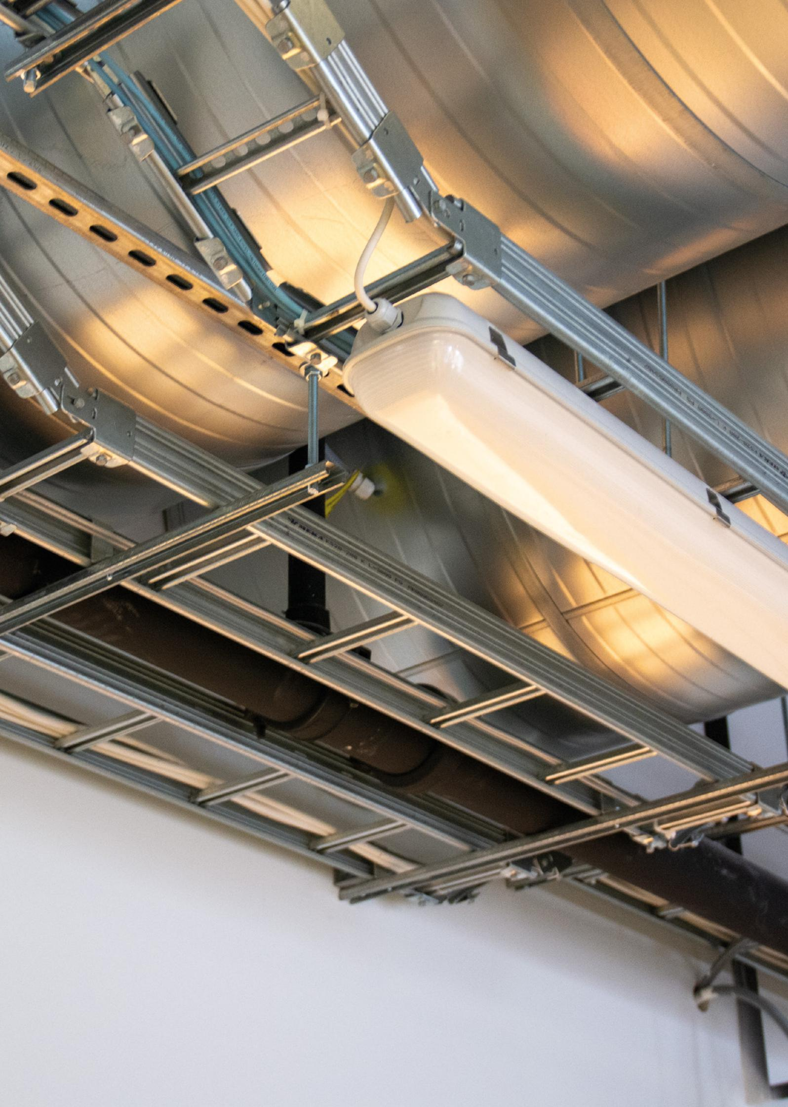
Covers KRL-KST are used to protect cables from damage, dirt and UV radiation as well as finishes the installation for KST pieces. If necessary, covers can be fixed with cover brackets KAP or screws. When using KAP covers are raised approx. 50 mm that adds cable space and improve better air flow.
